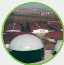
ANAEROBIC DIGESTION OF FOOD WASTE
